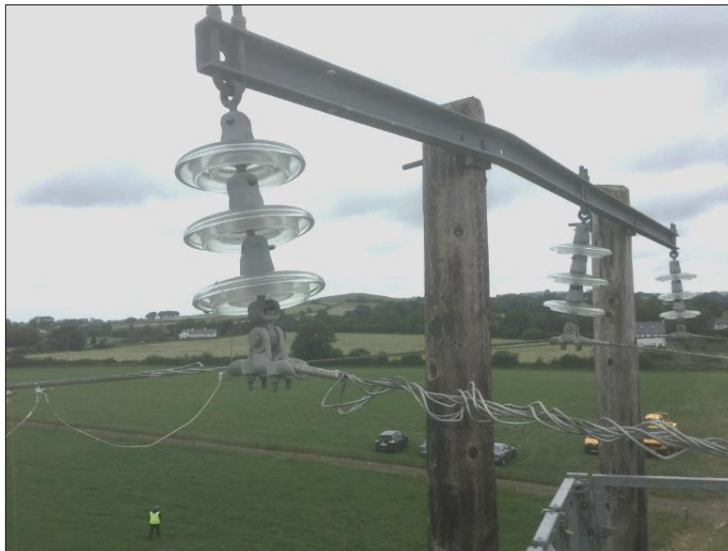
Photo No. 2: Damage to line and cross beam
